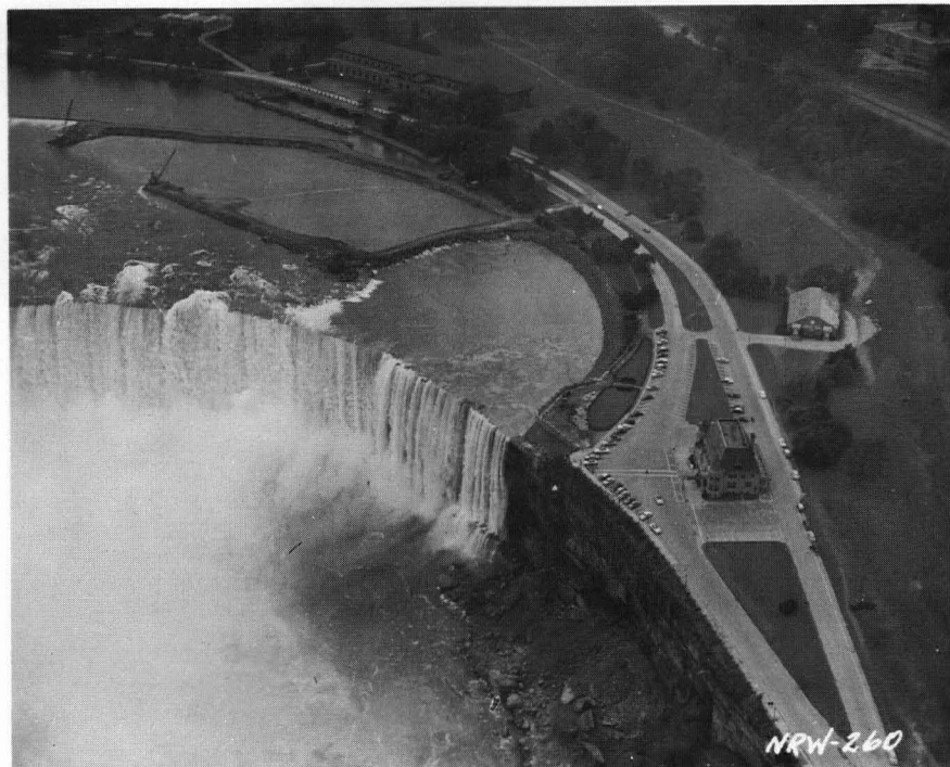
Photograph 17. Removal of cofferdam, Canadian end of Falls, 27 September, 1955.
