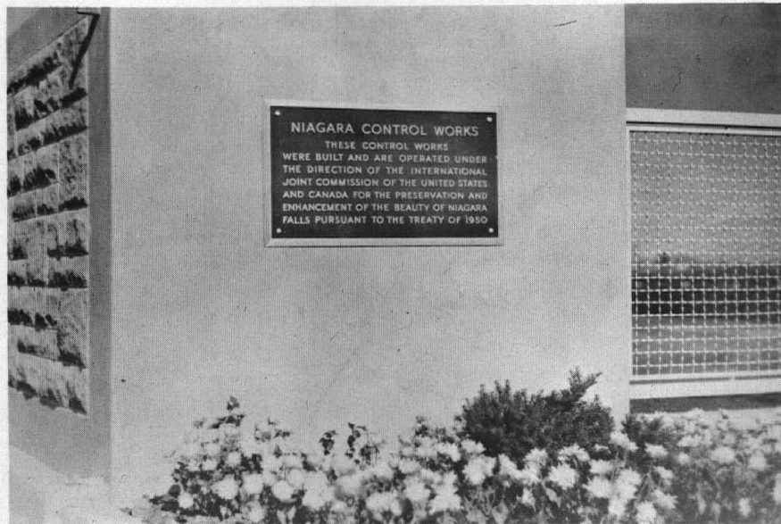
Photograph 23. Aluminum plaque on gatepost at control structure, 21 October, 1957.
