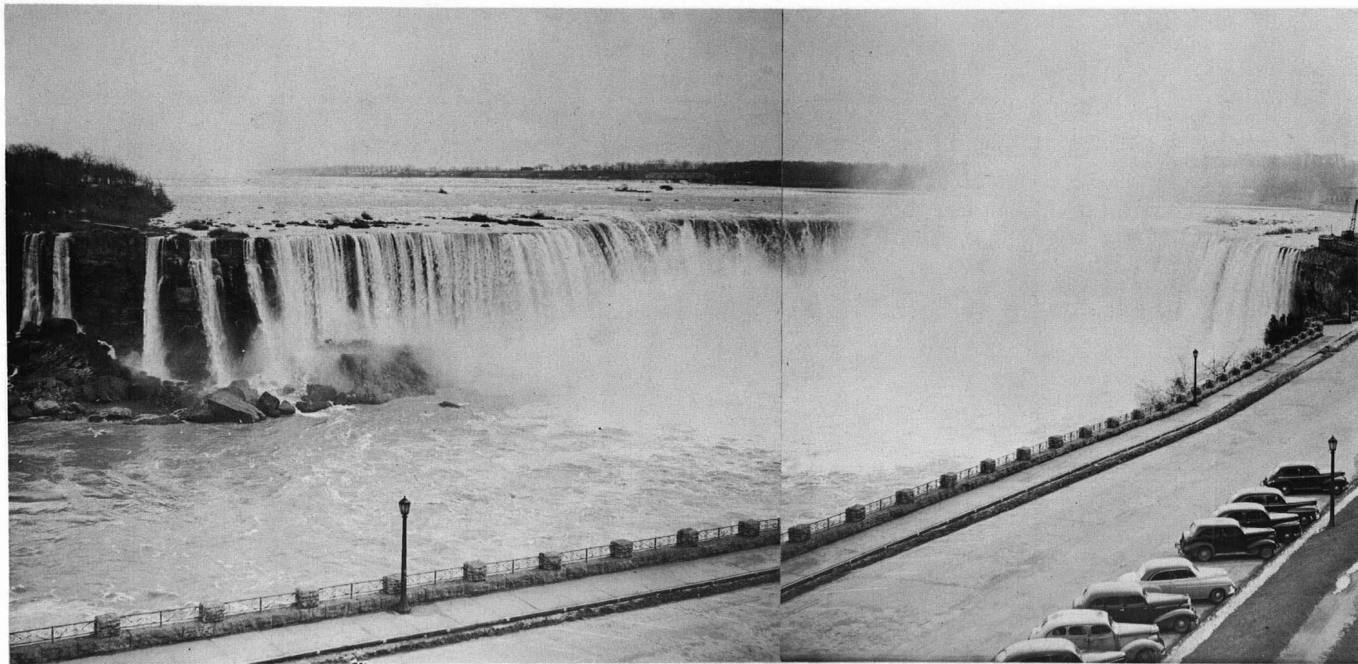
Photograph 20. Horseshoe Falls before remedial works, 5 December, 1950. Combined flow over Falls, 107,000 cfs.
