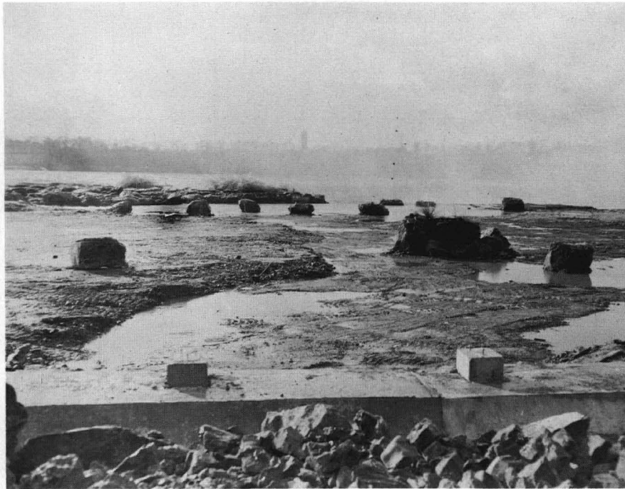
Photograph 14. Lower end of work area, Goat Island, 2 December, 1954.
