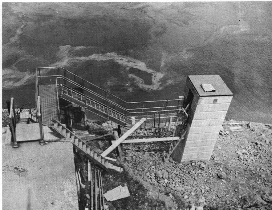
Photograph 21. Water level recording station, near foot of Ashland Avenue.
