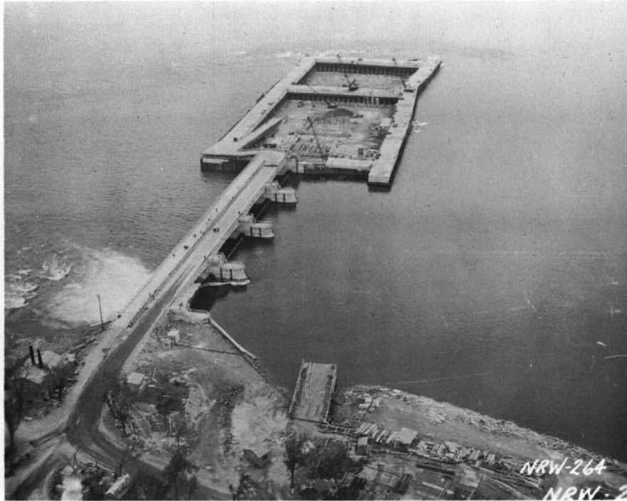
Photograph 3. First four gates in operation, stages 3 and 4 unwatered, control structure, 27 September, 1955.
