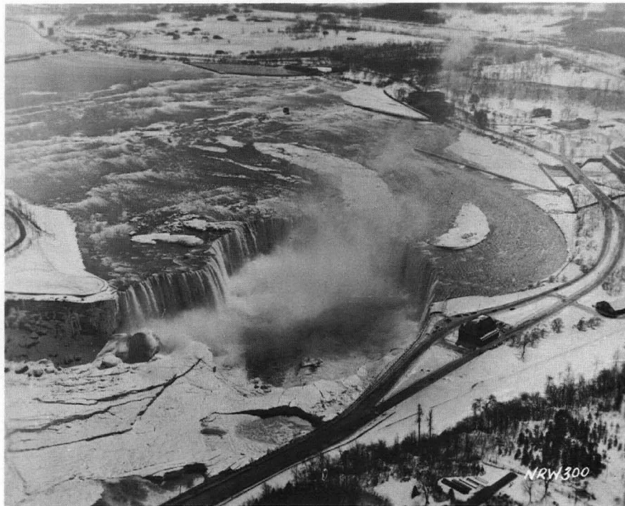
Photograph 19. Horseshoe Falls after remedial work, 19 March, 1956. Combined flow over Falls, 63,100 cfs.
