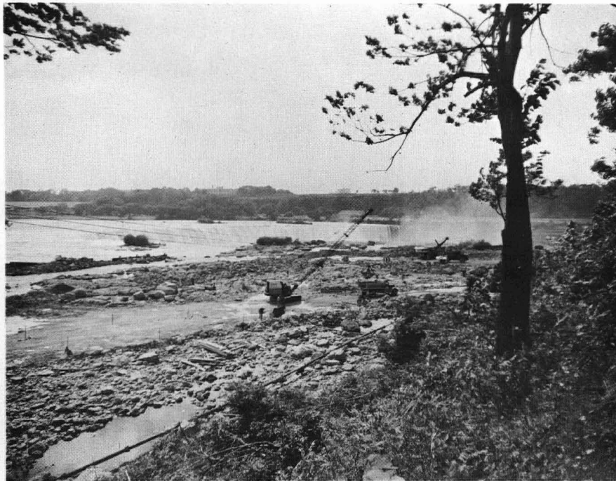
Photograph 12. Lower part of work area, Goat Island, 2 September, 1954.
