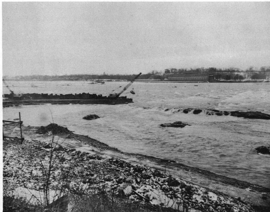
Photograph 15. Removing cofferdam, Goat Island, 16 December, 1954.
