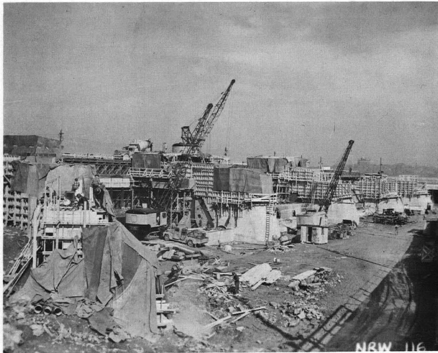
Photograph 2. Erection of piers for first four gates, control structure, 10 March, 1955
