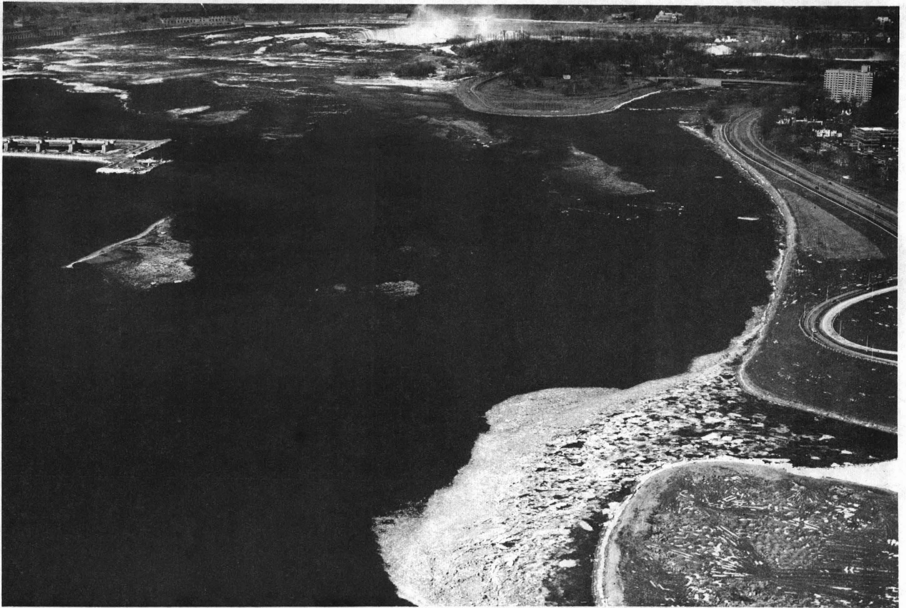
OBLIQUE AERIAL PHOTOGRAPH OF SHOAL AREA - MARCH 23, 1963 VIEW LOOKING DOWNSTREAM TOWARD GOAT ISLAND
